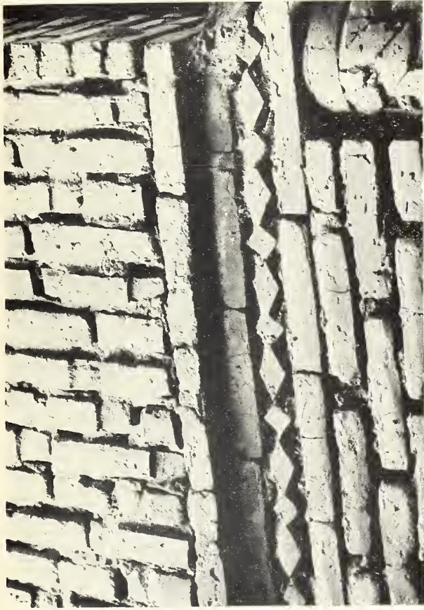
PHOTO. M. B. SMITH, NEG. L-150.34 FIG. 41—SANCTUARY, CORBELLED STILT OF WALL ARCH
